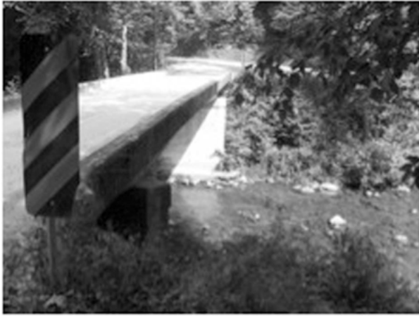
A bridge south of Mortimer
