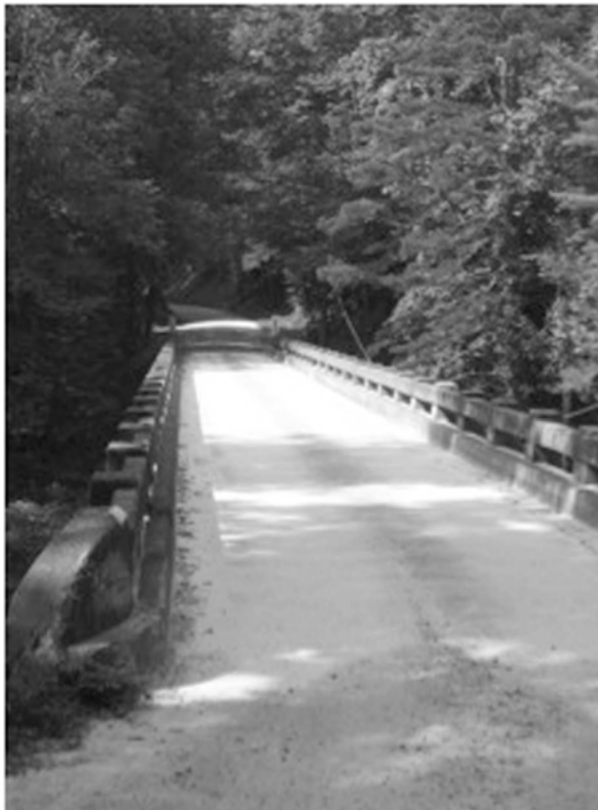
A lonely bridge north of Edgemont
